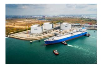
The SLNG terminal can receive, store, and regasify LNG shipped in by tankers from all around the world.
